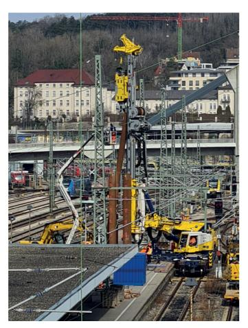
High-frequency vibration. The majority of sheet piles are vibrated into the soil using highfrequency vibrators. One particularly gentle method is hydraulic pressing of sheet piles. Diesel or hydraulic impact driving is primarily used in heavy soils and at a large distance from sensitive buildings.
