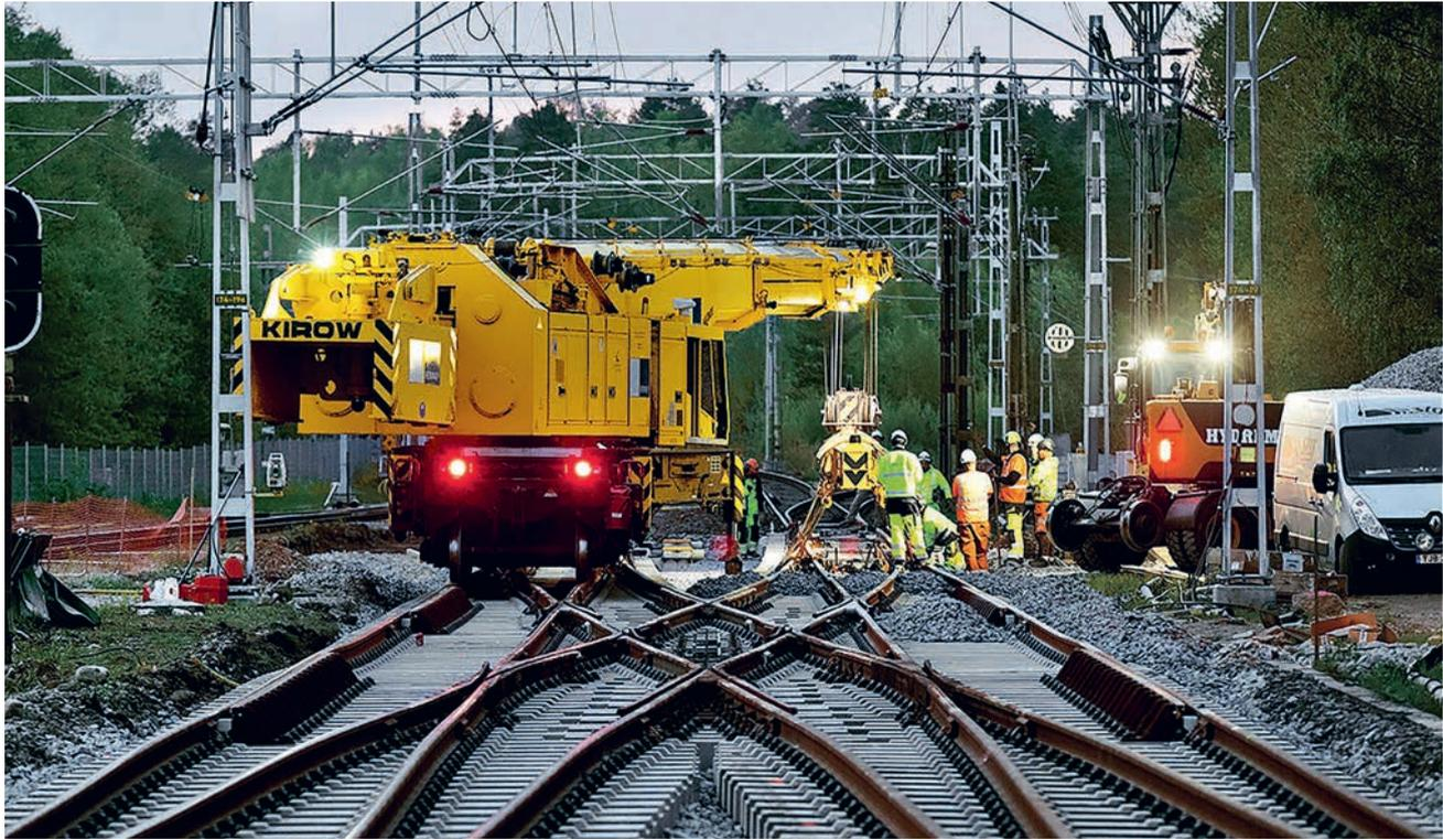
Green building site and environmentally-friendly installation of prefabricated components on the track
