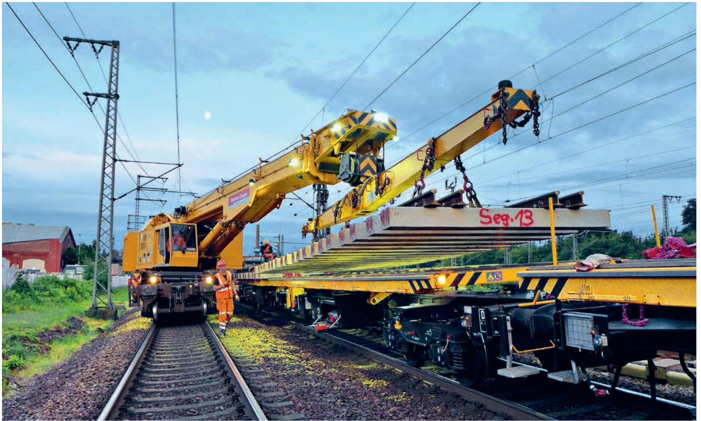
At the construction site, unloading can be performed at a convenient location for installation of the switch. The low height of the Switch Tilter's loading platform creates sufficient space for unloading under existing overhead lines.
