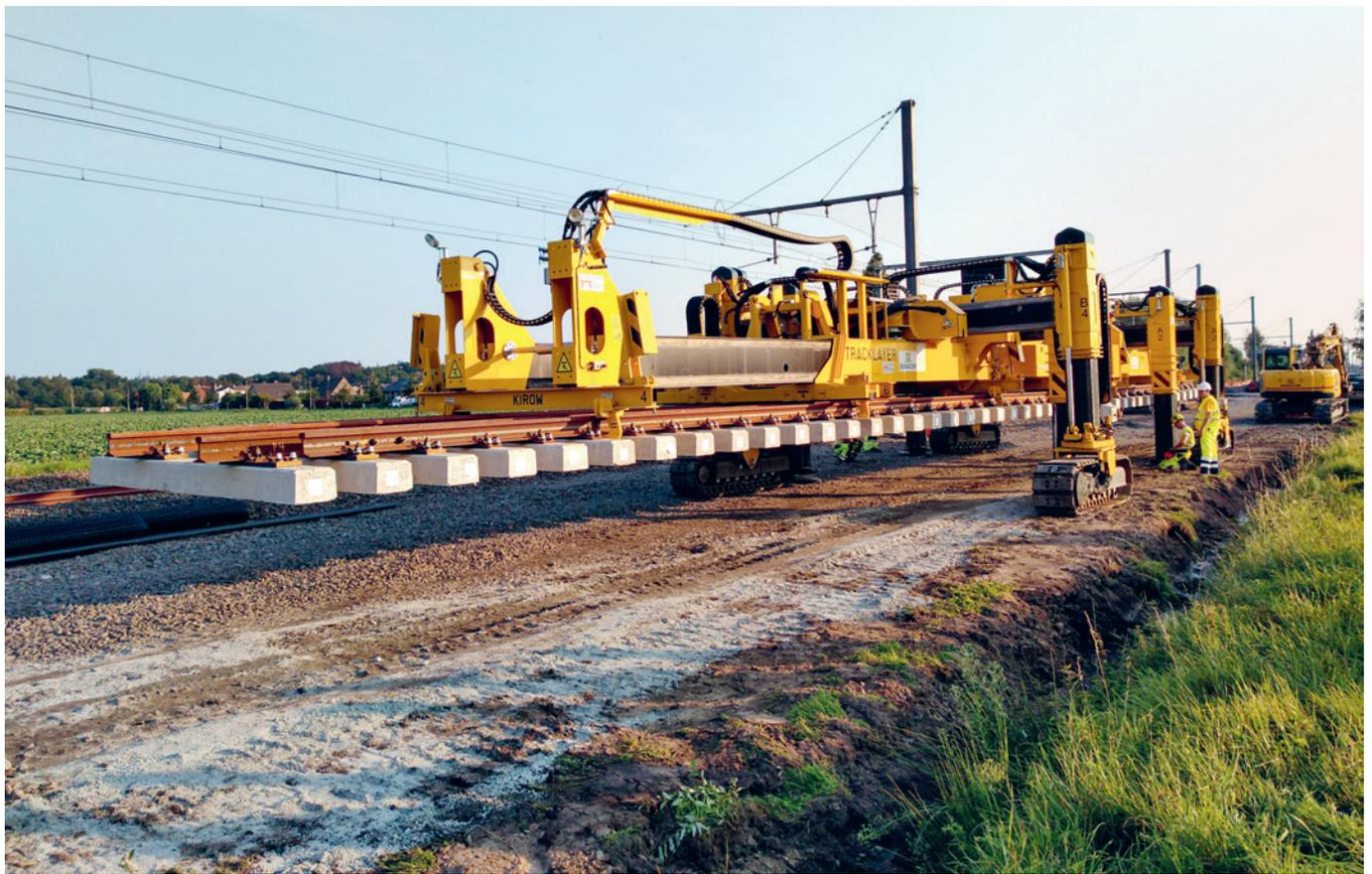
The Tracklayer is a multifunctional device for lifting, transporting and laying very long and heavy track and switch sections.
